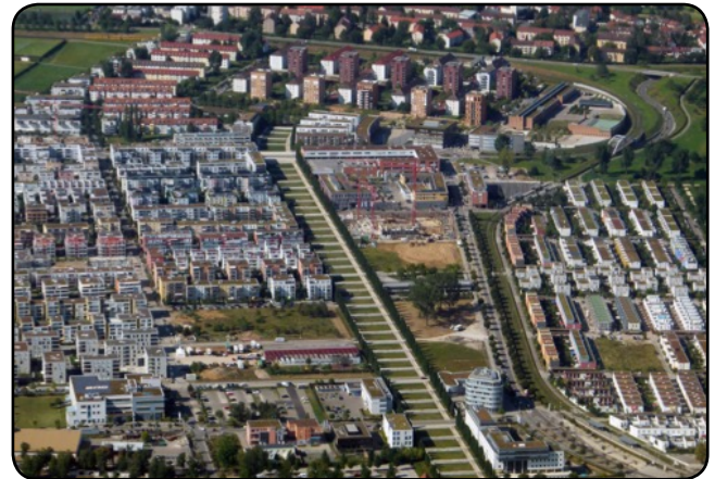
Figure 8. New development near Stuttgart, with no increase in stormwater runoff (Ramboll 2004).
